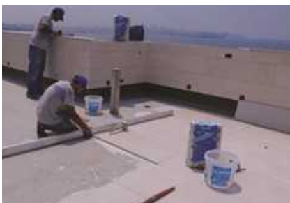
Tiling, painting, cornice installation...
