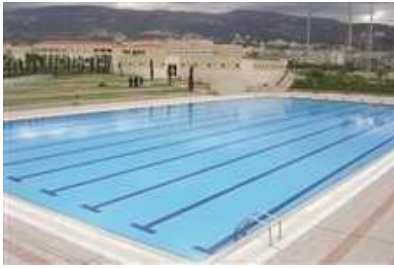
LEBANESE UNIVERSITY Waterproofing & swimming pool
