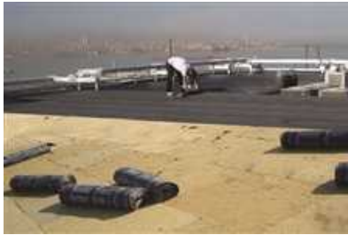
MTV Waterproofing & insulation
