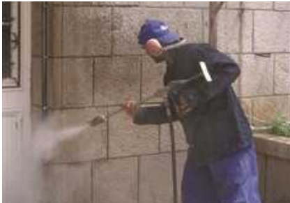
Water-jet cleaning, concrete repair, painting...
