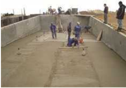
Plastering, screed, waterproofing, tiling &amp; grouting
