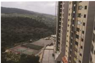
SKY TOWERS Waterproofing & sport court
