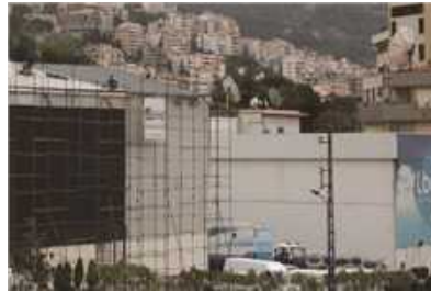
LBCI Waterproofing & insulation
