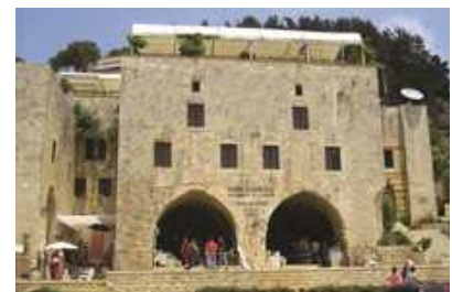
FAKHREDDINE PALACE Waterproofing
