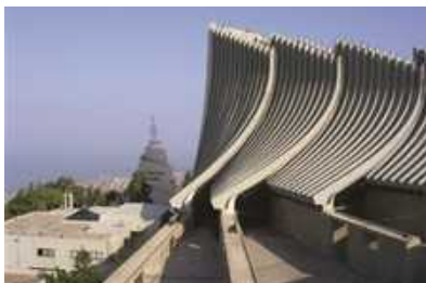
NOTRE DAME CATHEDRAL Waterproofing, concrete repair & paint
