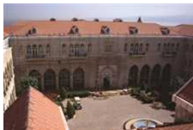
GRAND SERAIL Waterproofing
