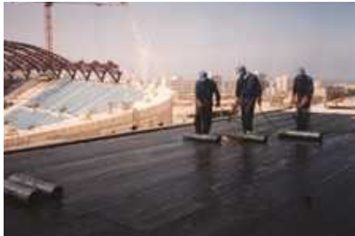
BEIRUT SPORT CITY Waterproofing & insulation
