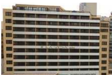
LA VIDA SUITE HOTEL Façade renovation
