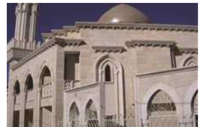
CHEHOUR MOSK Façade treatment
