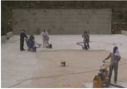
Surface preparation, coating, lining
