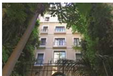
CONVIVIUM V Façade renovation
