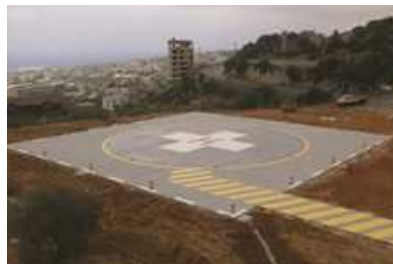
AL MAOUNAT HOSPITAL Helipad coating
