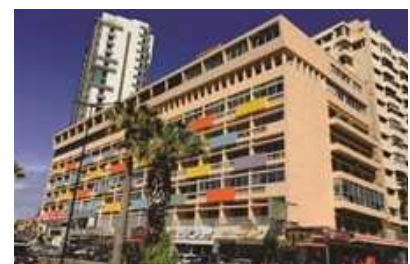
SHAMS BUILDING Façade renovation
