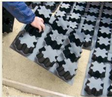
MOULDS ARE POSITIONED ONTO THE PREPARED SURFACE
