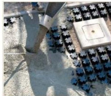
CONCRETE IS CAST, LEVEL WITH THE TOP OF THE MOULDS
