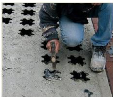
ONCE SET, THE TOPS OF THE MOULD ARE PUNCHED THROUGH AND CLEANED
