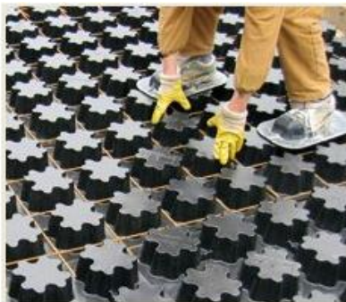
WIRE MESH IS PLACED ON THE SUPPORTS WITHIN THE MOULDS
